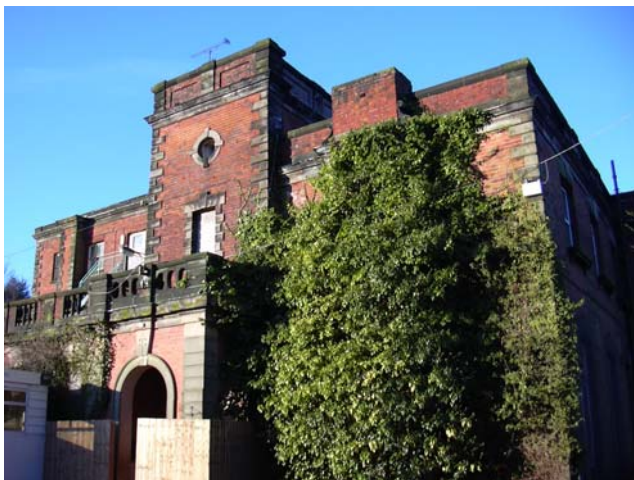
Photograph of the main building
