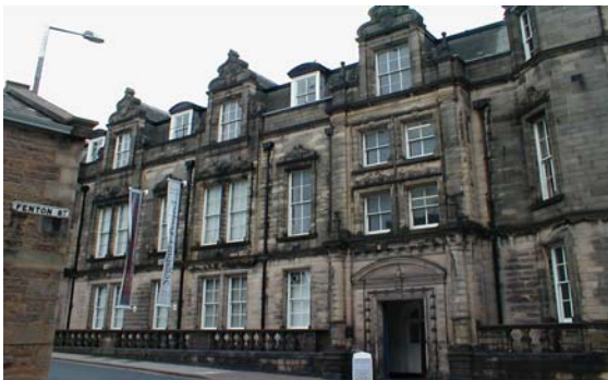
Photograph of the Building
