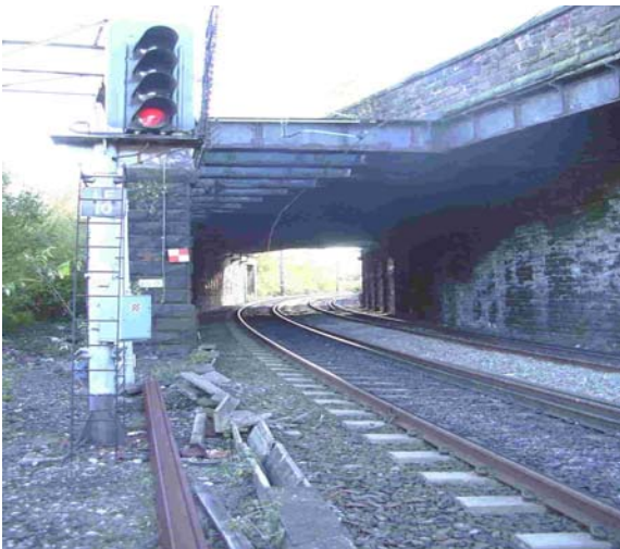
Picture of the Overbridge
